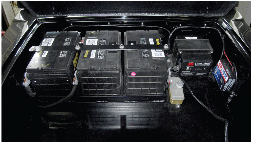
The charger included with this kit is the Quickcharger rated at 144 volts. It is a smart charger and runs through multiple charge cycles before turning off when batteries are full. (It is the small black box with the digital readout next to the batteries.) The CarQuest Smart Battery Charger is for the 12 vdc accessory battery, which powers a separate 12-volt system which runs the lights, turn signals, horn, and radio.
